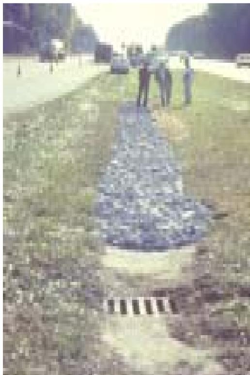
**Plate 8-1: Infiltration trench
