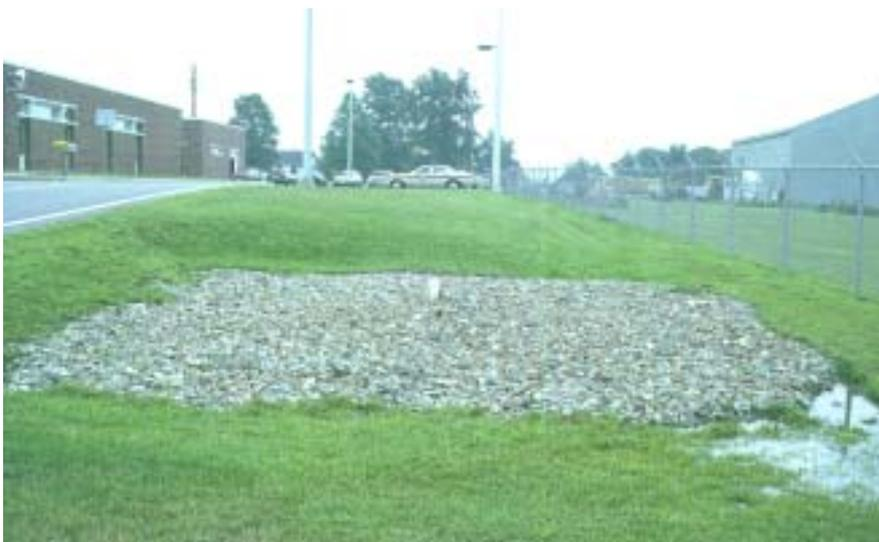
**Plate 8-2: Infiltration trench with a swale for pretreatment**
