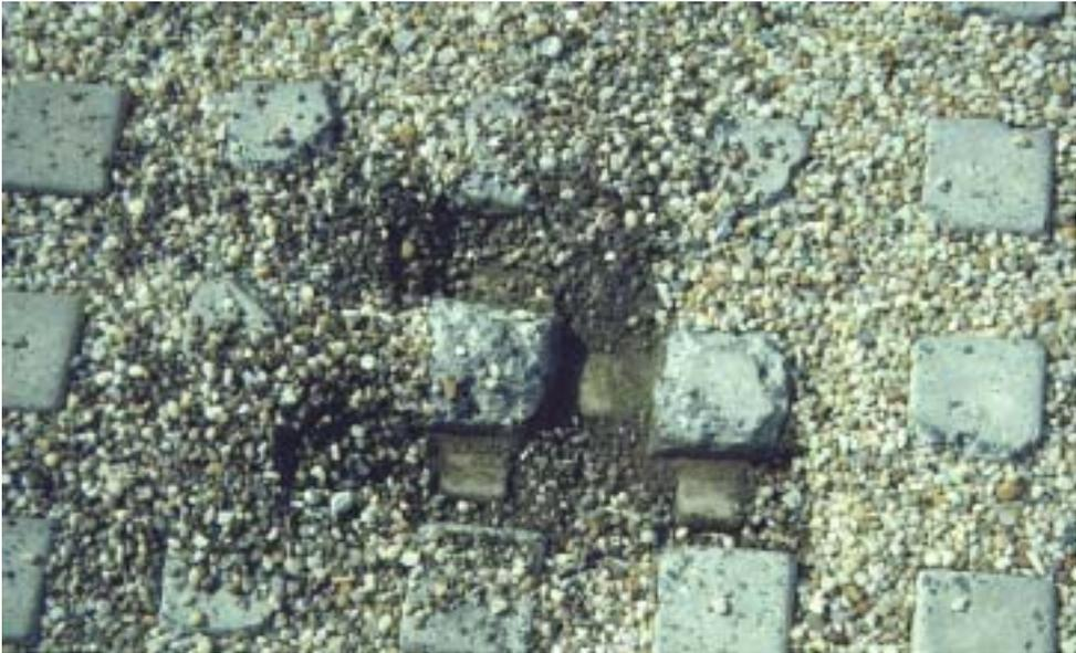
**Plate 8-7: Modular paving with pea gravel filler**
