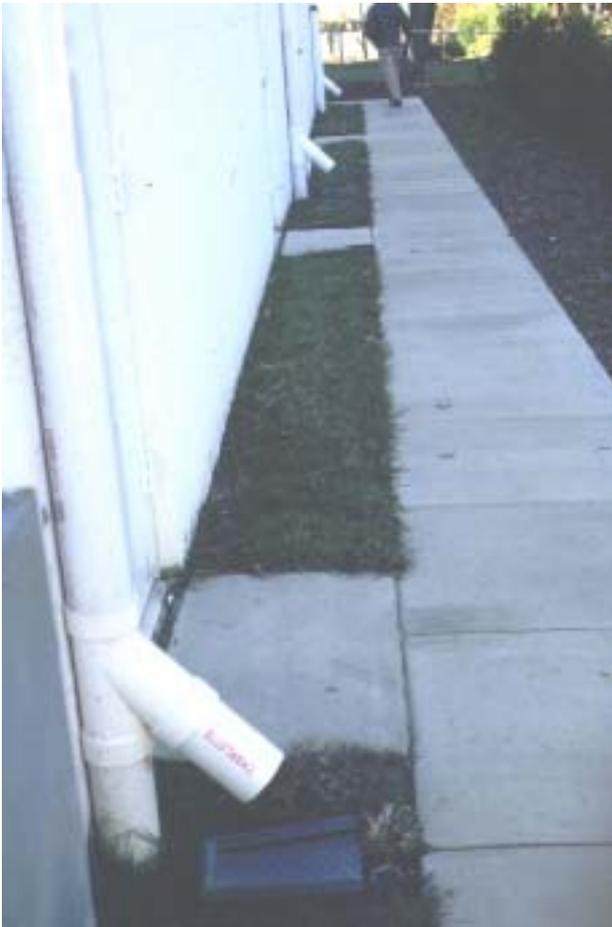
**Plate 8-4: Infiltration dry well**
