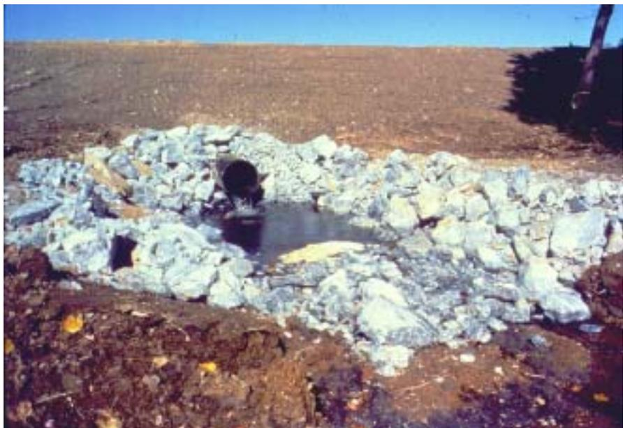
**Plate 13-1: Example of riprap at a stormwater outfall**
