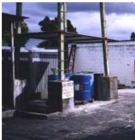
Plate 3-1: Chemical roof and bunding
