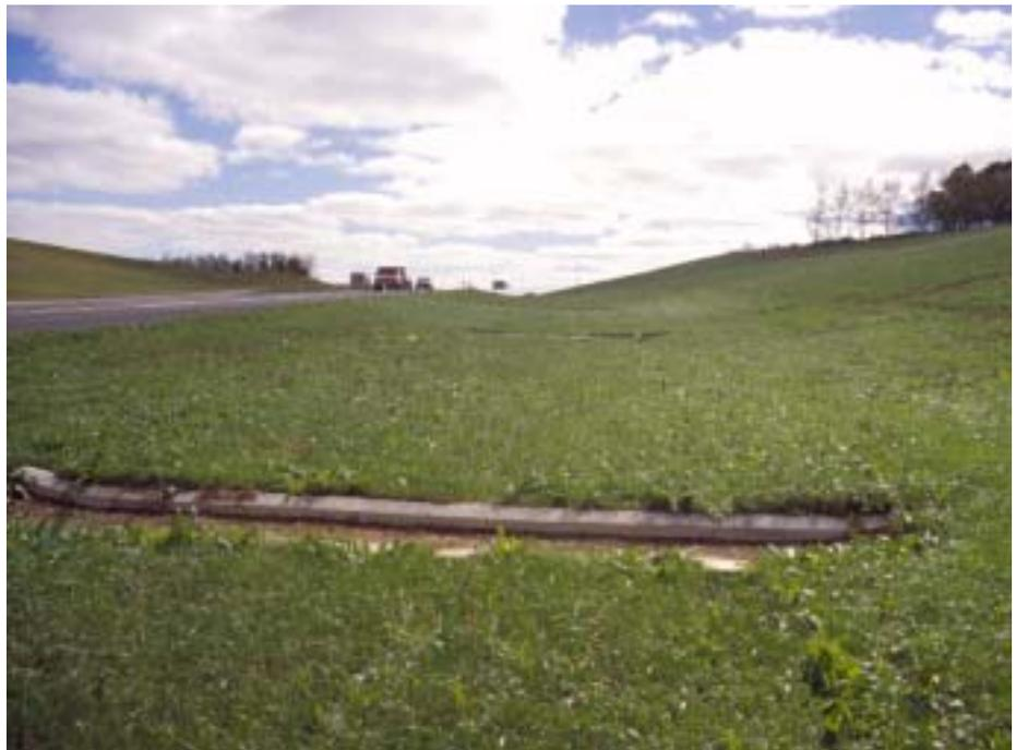
**Plate 9-4: Swale level spreader to maintain dispersed flow in swale bottom**
