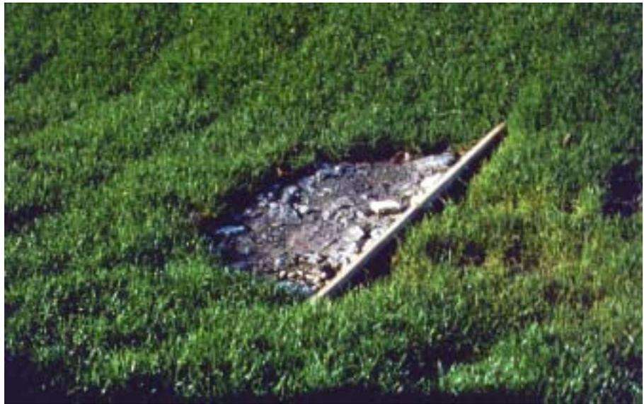
**Plate 9-3: Detail of a swale check dam**
