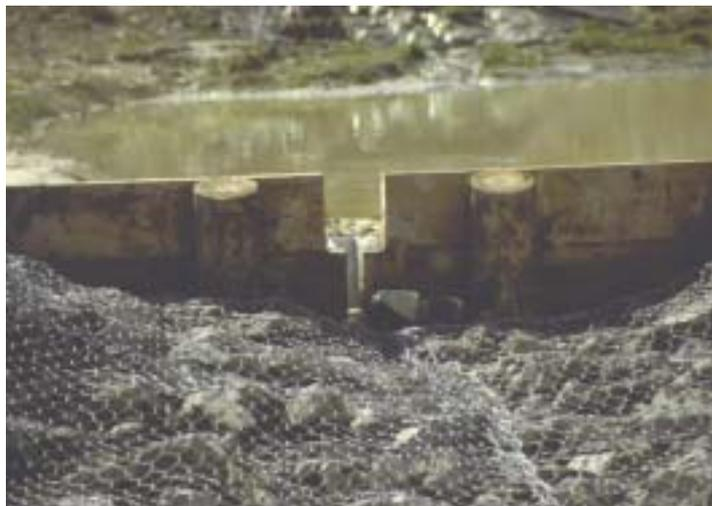
**Plate 5-3: Outlet Structure Showing Multiple Storm**
