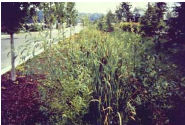
length-to-width ratio of 5:1 must be provided. The minimum swale length remains at 30 metres.
